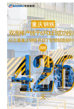
At 14:00 on June 30, 2021, the Double HSD System for Chongqing Iron & Steel production line was put into operation after 426 days of construction, marking the beginning of a new era of intelligent manufacturing for the Company.
